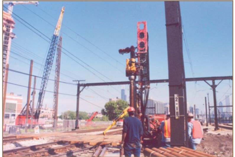
18th Street Pedestrian Bridge - 100 ton micropiles, 90 ton driven piles.
